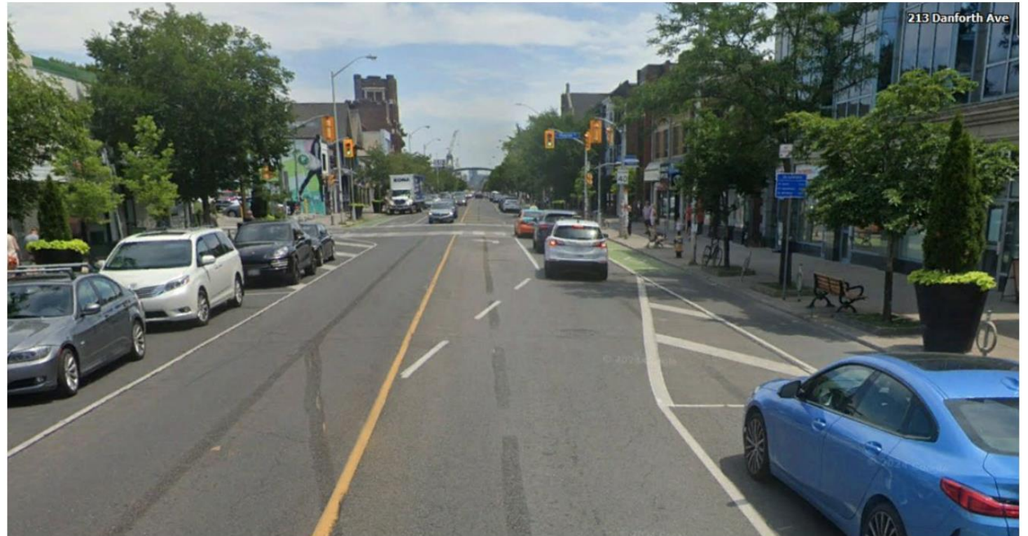
Figure 5.20: A shorter and more abrupt turn lane taper used on Danforth Avenue (40 km/h posted limit) in Toronto
