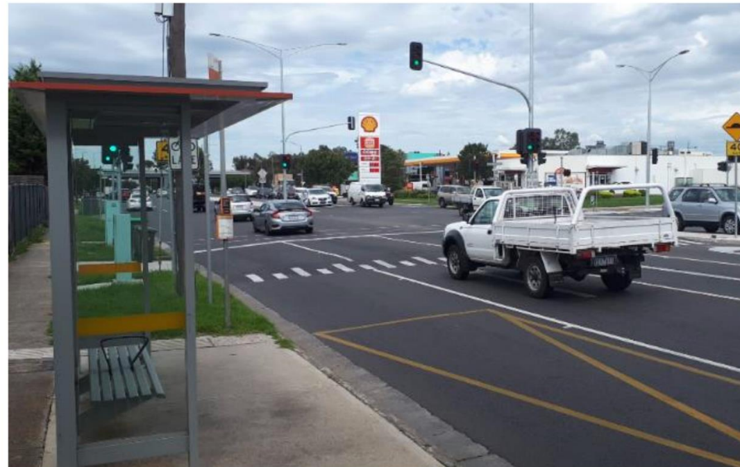
Figure 5.2: Raised safety platforms on Dalton Road, Thomastown, Melbourne
