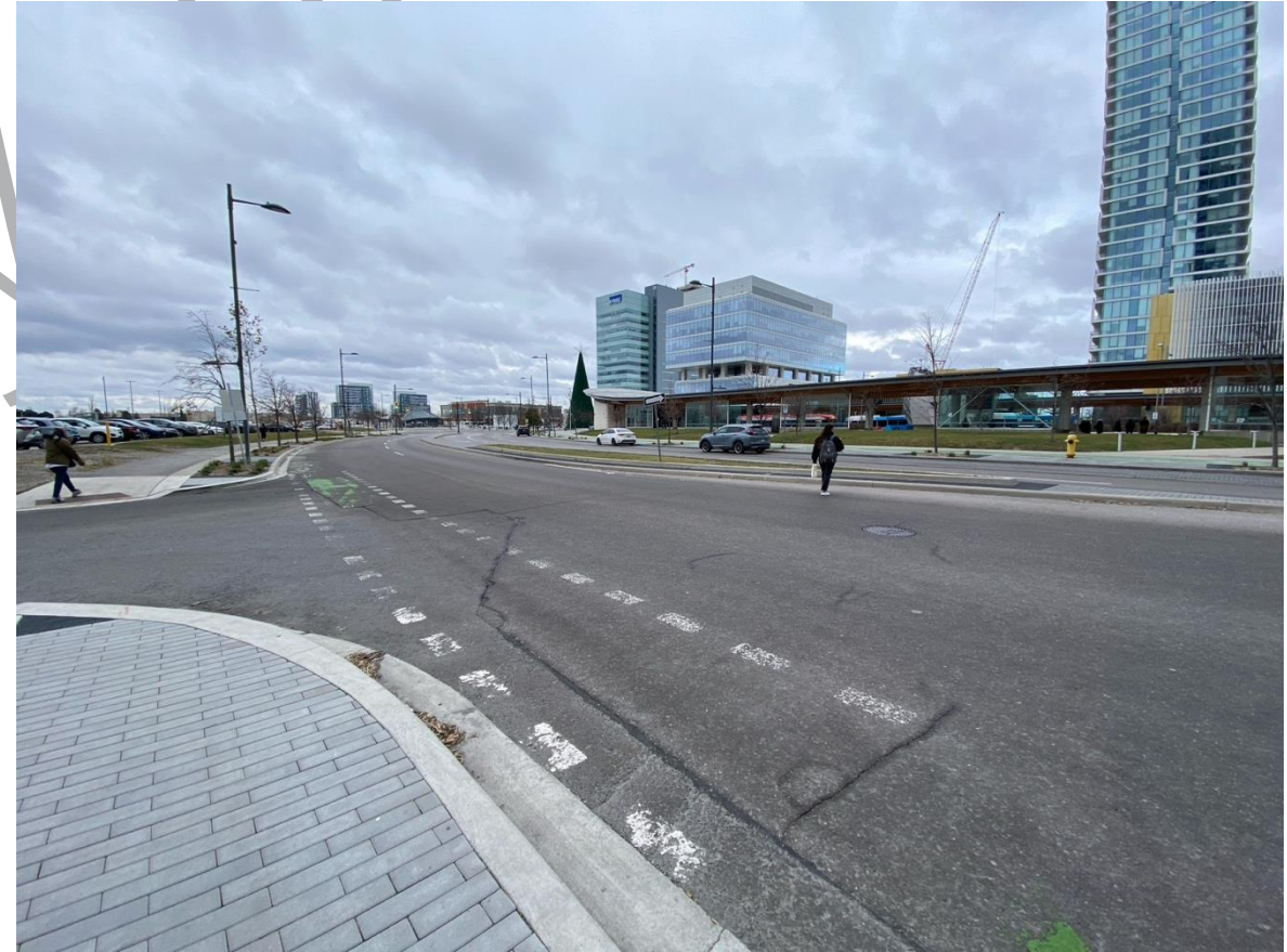
Multi-Lane Avenue in Vaughan (Mobycon)
