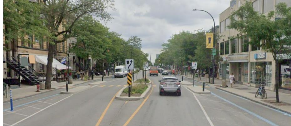
Figure 6.10: Saint Denis Street treatments (left to right): Pedestrian refuge island, island bus stop, bump outs
