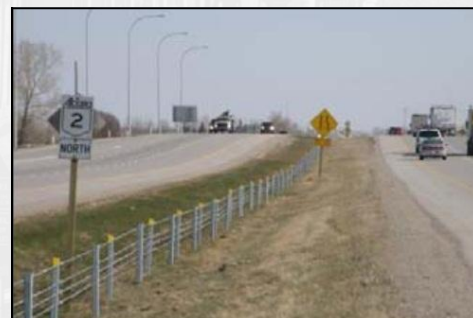
High-tension cable median barrier
