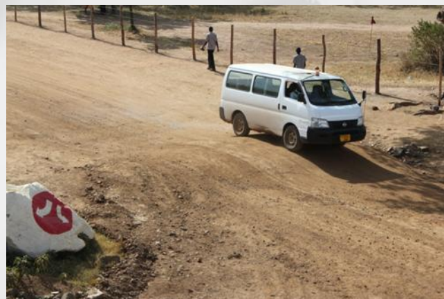
Speed humps made of 'dirt' have been used to slow traffic.
