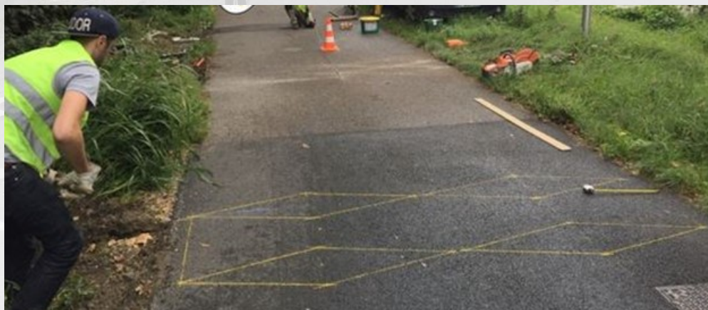
Figure 2: Inductive loops being installed on a multi-use pathway to count bicyclists
