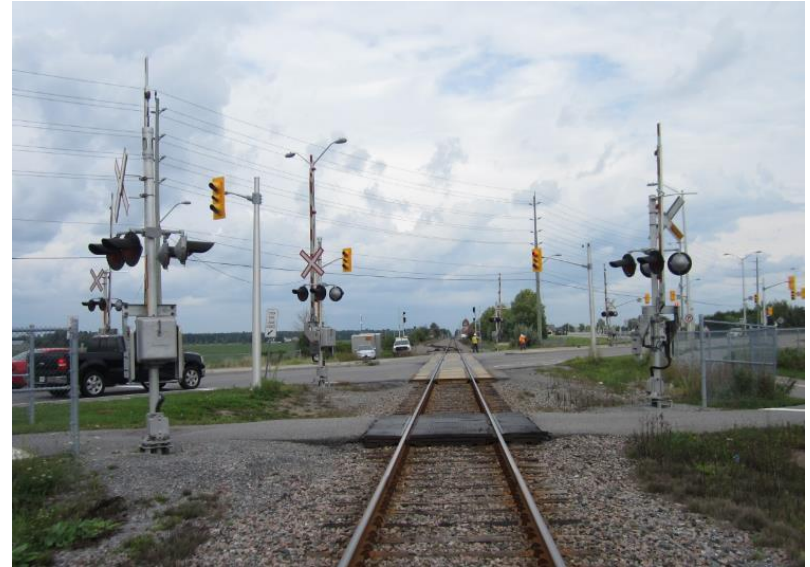
Crossing with a walkway/path/trail
