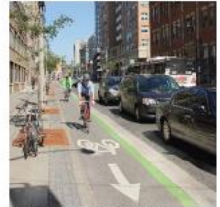
Raised Cycling Facilities
