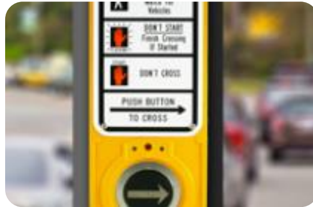
Accessible Pedestrian Signals
