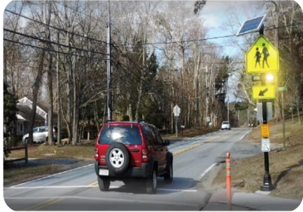
New Rapid Flashing Beacons at Crosswalks
