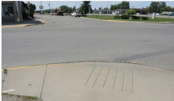
Orientation of the curb ramps
