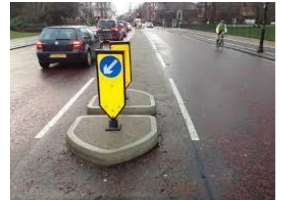
Traffic Islands: narrow the road and reduce the speed of passing traffic
